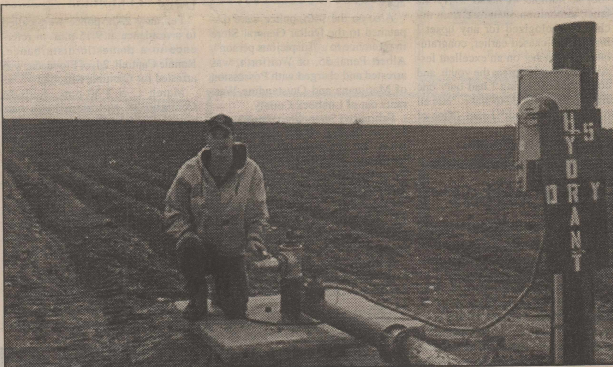
FLOYDADA VOLUNTEER FIREMAN JASON PYLE kneels by one of 25 dry hydrants that the Floydada Volunteer Fire Department, in cooperation with land owners/operators, have installed. These dry hydrants are located throughout the part of Floyd County that the Floydada Volunteer Fire Department protects. The dry hydrants are connected to a landowners existing irrigation well and can provide quicker access to firemen out in the county fighting structure or CRP fires. "It will save us a lot of time in case we run out of water," said Jason. "We won't have to run 10 miles back to town to fill up the water truck." Funds for the purchase of the materials were provided by a grant from the Texas Forest Service through the Floyd County Commissioners Court. Because the firemen did the work themselves, at a fraction of the cost, they were able to use the grant money to put in more wells than expected. Staff Photo
