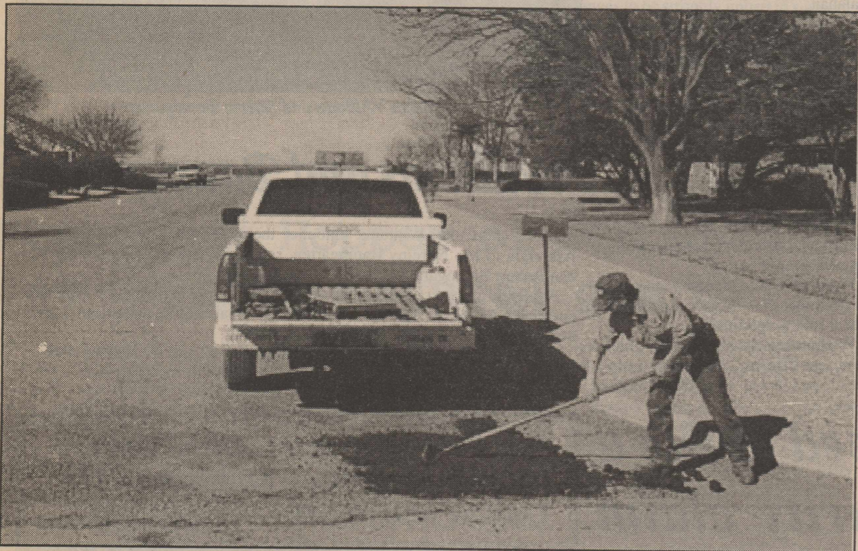
FILLING THE POT HOLES-Floydada City employee Gerald DeLeon is shown in the 900 block of W. Kentucky patching one of the many pot holes around town caused by the recent ice storm. Staff Photo
