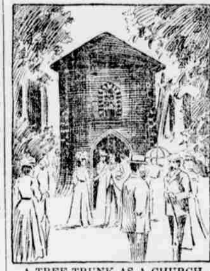
A TREE-TRUNK AS A CHURCH. trees in Gippsland, Victoria, was felled at a distance of twenty feet from the ground. The wood of these trees is very soft when growing, and when newly cut down, but hardens when it is dead. In this tree, while the wood was still soft, the stump was hollowed out, openings for doors and windows were cut, and a roof was placed upon it. In this way a room was formed, said to be twenty-five feet in breadth, and capable of accommodating fifty people. Religious services have frequently been held there, the people for miles around assembling out of curiosity; but this curiosity has led to blessing, and a movement is now on foot for erecting a substantial church.
