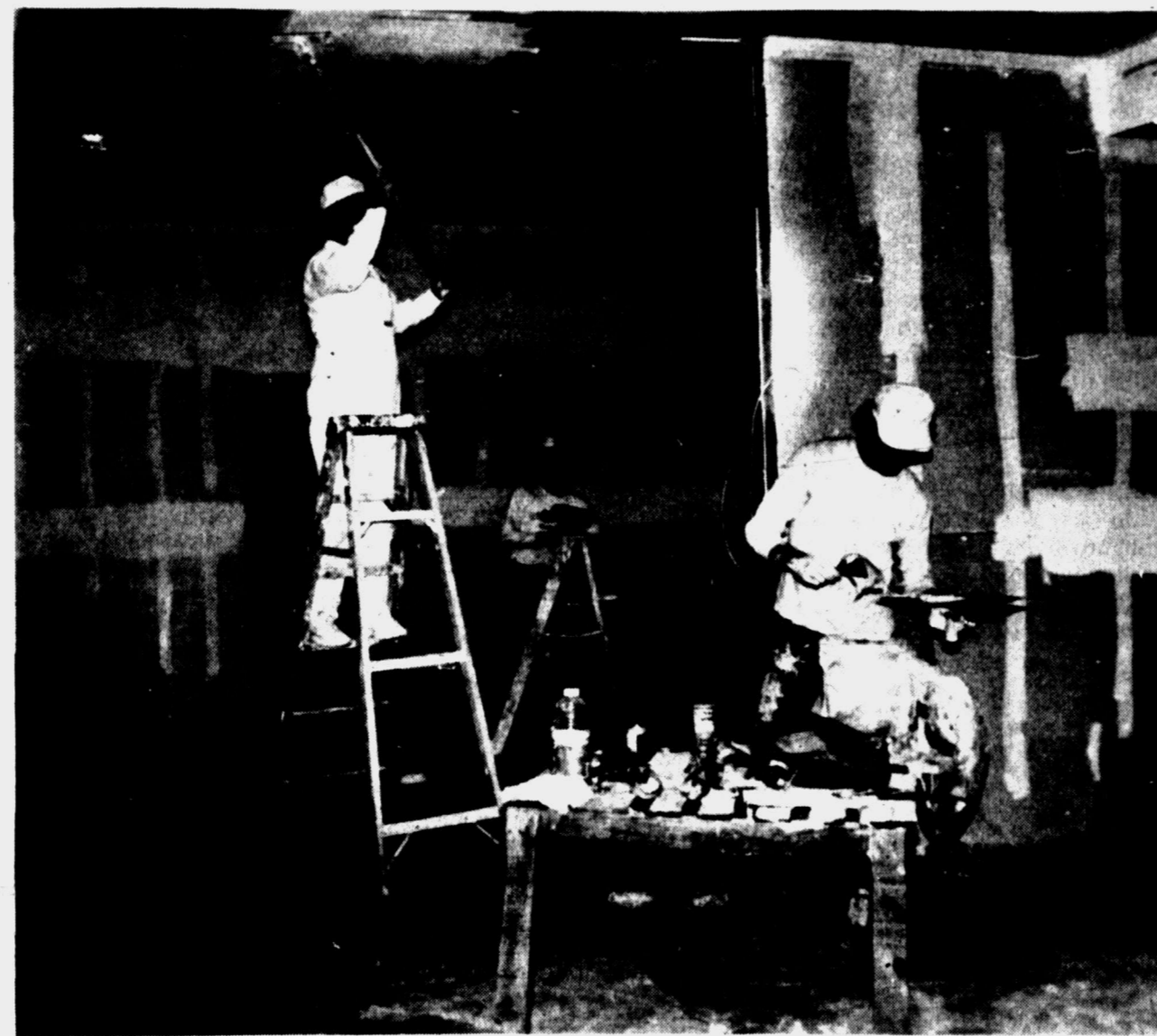
NEW CONSTRUCTION — Ronnie Woolridge, Cornell Davis and Billy Roach, from left, Snyder since January, 1994. (SDN Staff Photo) prepare the ceilings and walls for paint and texture in one of the 12 new homes constructed in the 1900 block of 30th Street and College Avenue.
