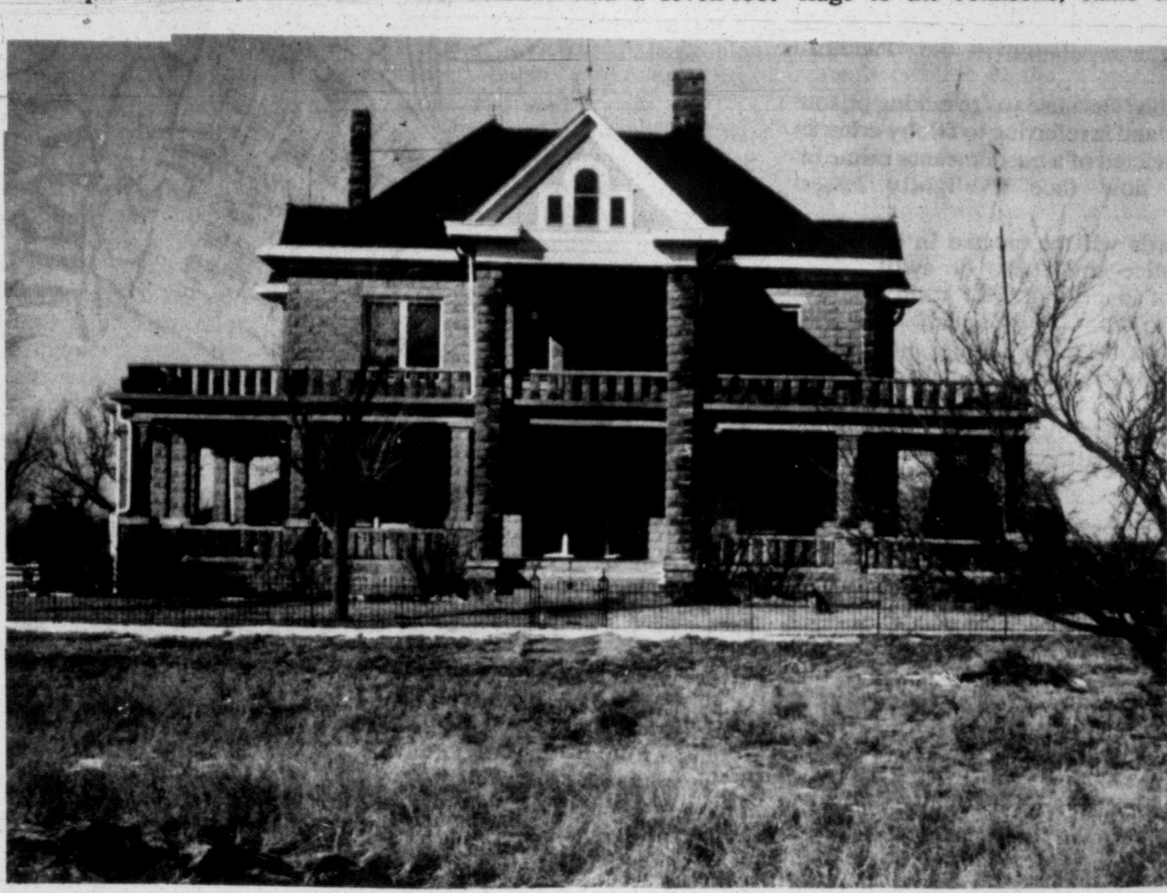
JOHNSON HOUSE — Mr. and Mrs W.A. Johnson built this beautiful 16-room house for their family home in 1910. The cement blocks used in its construction were made from sand and gravel on the premises. To ensure that the mix was cor-
