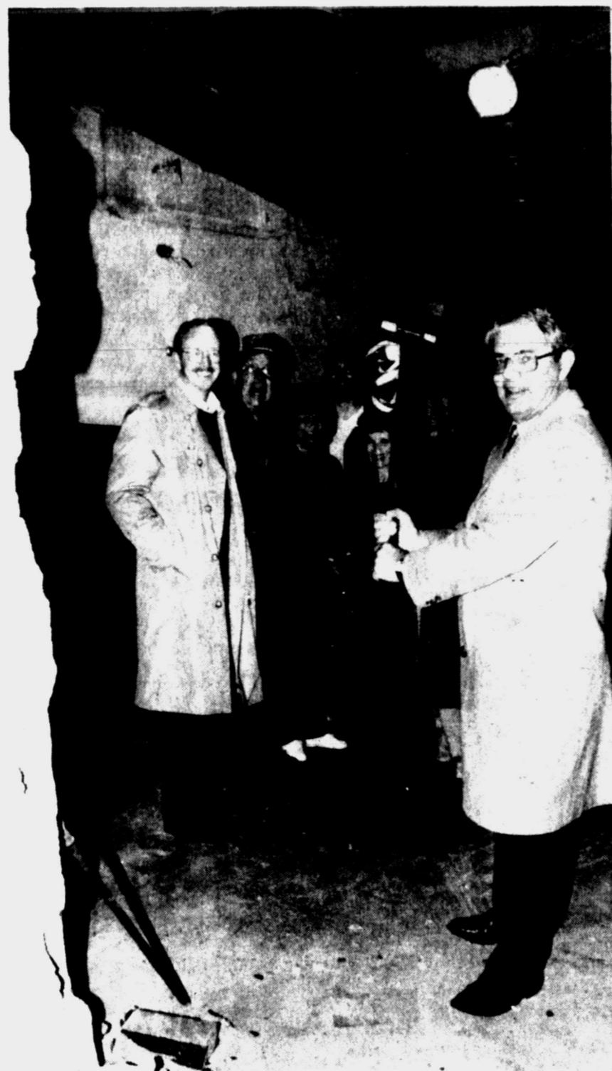
SWINGING THE HAMMER — John Fenton, president of the Ritz Theatre board of governors, gets ready to swing a sledge hammer Saturday morning to mark the beginning of the renovation of the inside of the Ritz Theatre. The exterior renovation has been completed and plans are to have the theatre functional by this fall. (SDN Staff Photo by Wade Warren)
