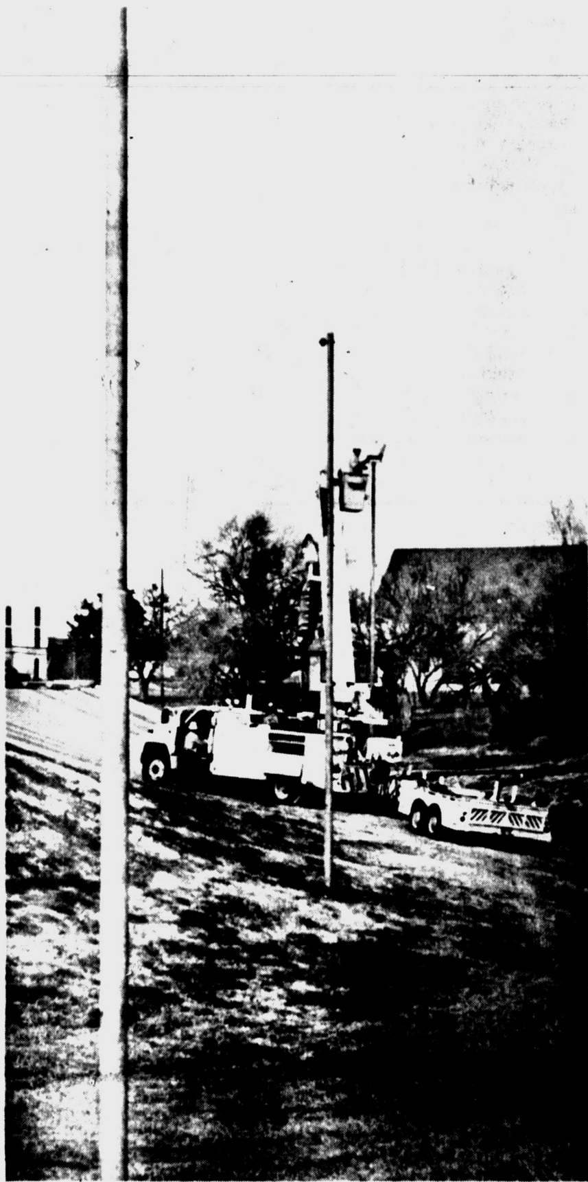
DEEP CREEK LIGHTS — TU Electric crews are currently installing lights along portions of the walking trail at Deep Creek. This portion of the trail is from 30th Street to College Avenue and includes the parking area on College Avenue. (SDN Staff Photo)
