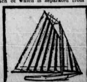
ropes are connected to the after corner of the lower end of each section and there are guiding leads for the ropes. A mainsail constructed in this fashion was tested recently, and it is said to at it proved more serviceable in various respects than an old-fash-ioned mainsail. The main advantage claimed for this new sail, however, a said to lie in the fact that it enables a yachtsman to utilize to the uti even a slight breeze.
