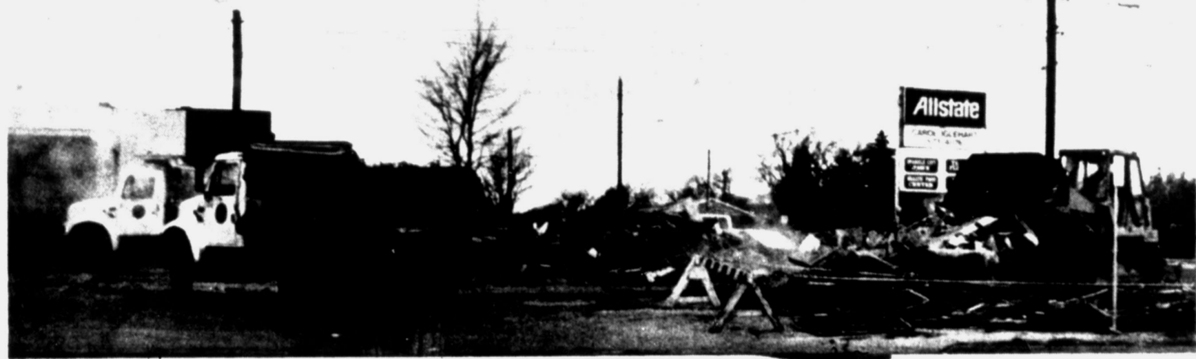
CLEANING UP — City crews were busy before the holidays demolishing an old service station located on the southwest corner of the intersection of 37th Street and College Avenue. City officials
