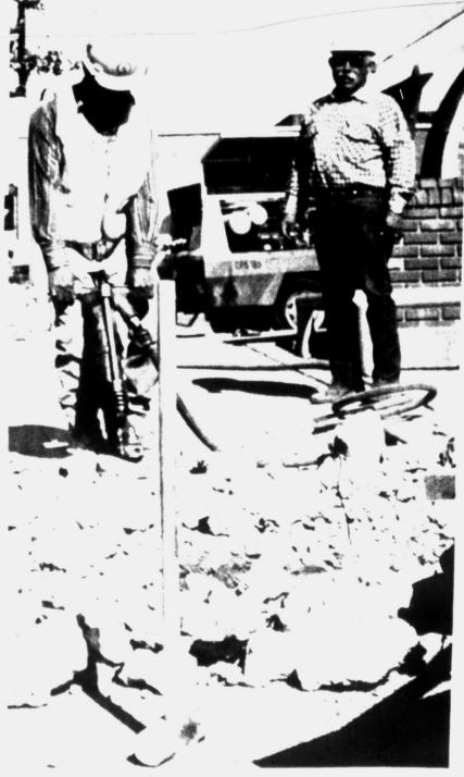
EASIER ACCESS — Crews with the Texas Department of Transportation have been busy around Snyder lately as they have been installing wheelchair ramps at the end of sidewalks which are on the state's right-of-way. Alyandro Ruralas operates a jackhammer in preparing one of the ramps while Otillio Rodriguez observes. (SDN Staff Photo)
