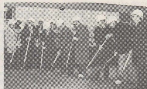
NOV. 29 GROUNDBREAKING . . . AND CONSTRUCTION MOVES AHEAD
