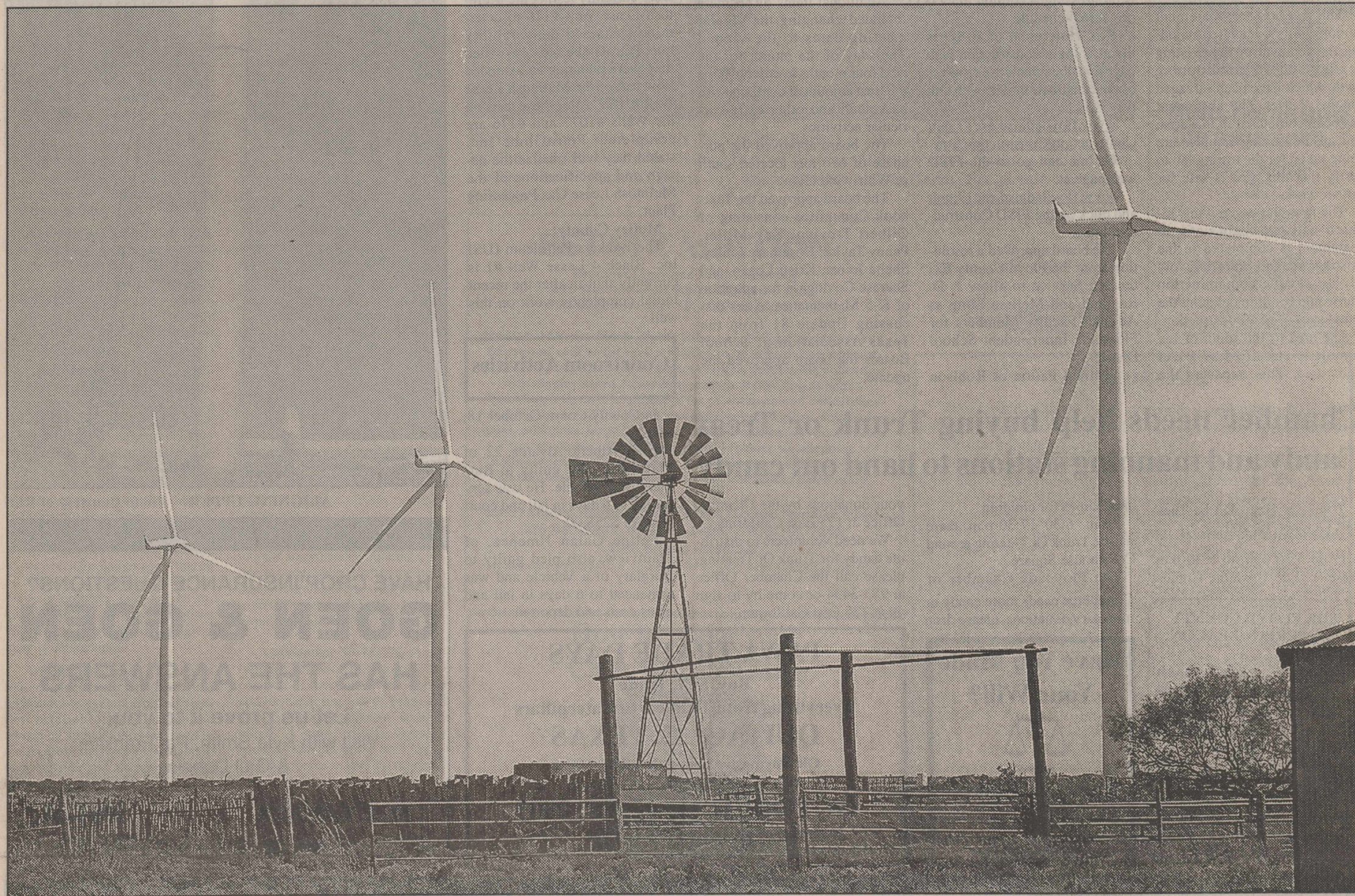
OLD AND NEW--This photo was taken by Al Jensen, RES Project Manager, at the Muncy Ranch site where wind turbines are being placed. Jensen was struck by the view of the old windmill sitting between the new wind turbines. RES has erected 8 turbines so far, but the project has been stopped because of high winds in the County this past week. According to workers at the site, the cranes cannot lift if the wind is over 23 mph.
