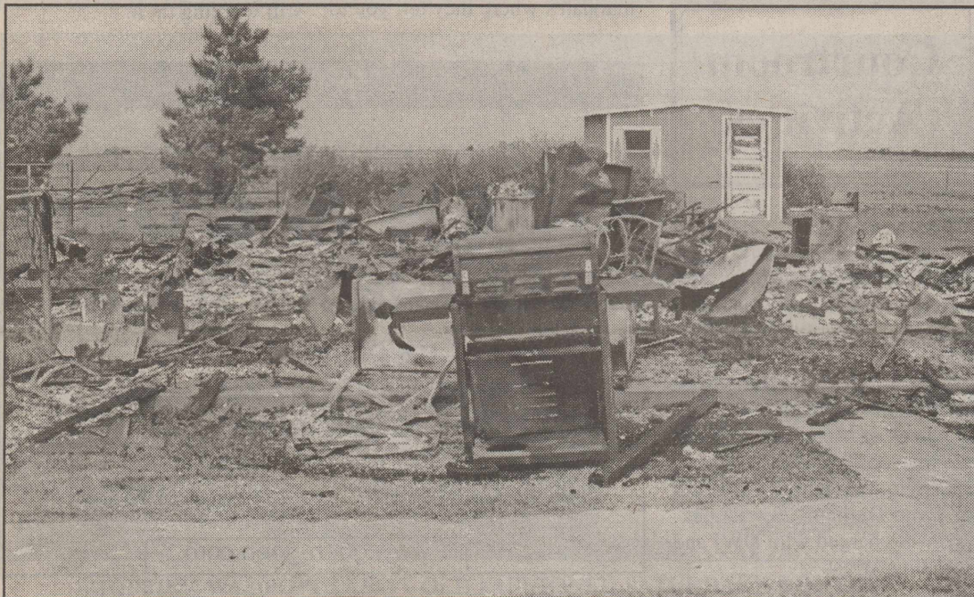
CHARRED REMAINS of a 2 bedroom home are all that is left for the Castillo family. The home, located almost one mile west of Floydada on the Sandhill Hwy, burned down September 11th. Staff Photo
