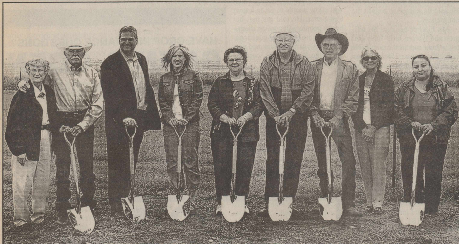
LANDOWNERS OFFICIALLY BREAKING GROUND ON THE RES WIND TURBINE PROJECT WERE: (l-r) Edith and Norman Muncy, RES Americas President Craig Mataczynski, Shanna Bain Pritchard, Edwina and Ron Davenport, Raz and Kay Ware, and Floydada Chamber of Commerce Manager Patti Sanchez. Courtesy Photo
