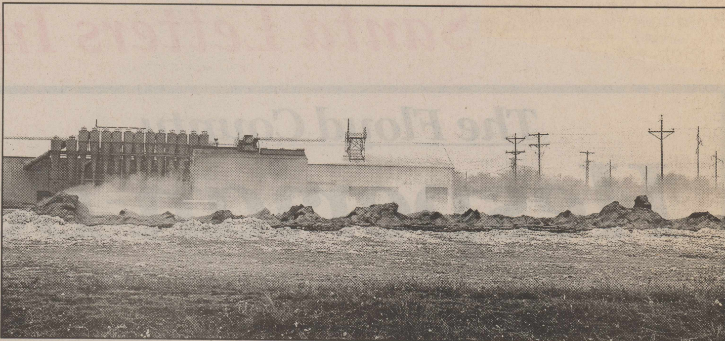
REMAINS OF 22 COTTON MODULES DESTROYED BY FIRE SUNDAY NIGHT -According to City Manager Gary Brown, the fire that destroyed 22 cotton modules at the Floydada Coop Gin is still under investigation. "The starting of the fire is listed as suspicious," said Brown. Floydada Fire Chief Carroll Sims said, "One fire truck pumper and three brush rigs, with volunteer fire fighters, were on the scene around 4:30 p.m. Sunday. We were fighting the fire until around 9 p.m. Sunday night. Several modules were burning at the same time when we arrived." Staff Photo
