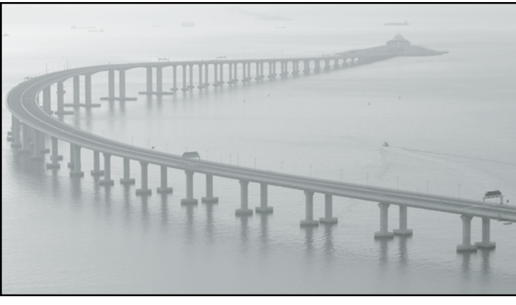
The Hong Kong-Zhuhai-Macau Bridge is seen in Hong Kong, Monday, Oct. 22, 2018. The bridge is the world's longest cross-sea project, which has a total length of 55 kilometers (34 miles).
