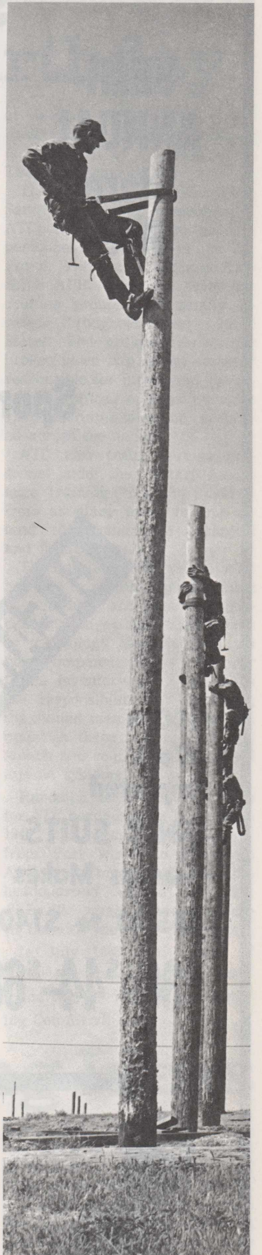
Students of the Electrical Distribution Systems, Installation and Maintenance Course at the Sheppard Technical Training Center, Sheppard AFB, Tex., must become skilled pole climbers to successfully perform their jobs. The 13-week course is designed to train students to construct and maintain electrical systems conducting as much as 15,000 volts of electricity. (USAF PHOTO)
