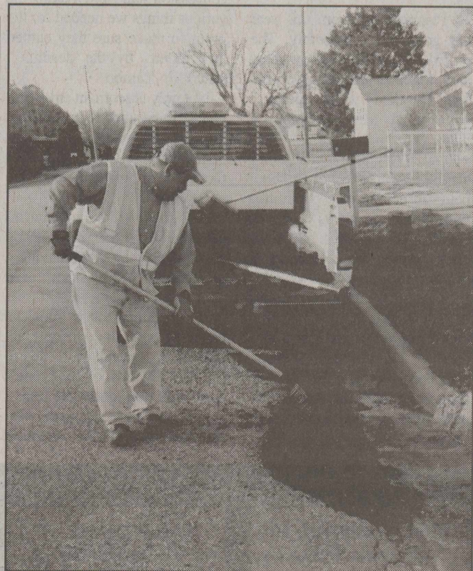
Courtesy Photo Floydada City employee Eddy Sanchez fixes potholes caused by recent rainfall.
