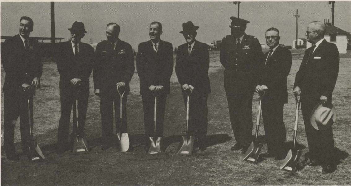
GROUND-BREAKERS — Reese and Lubbock officials joined in breaking ground for construction of the new 3500th Pilot Training Squadron operations building Monday. Lined up ready
