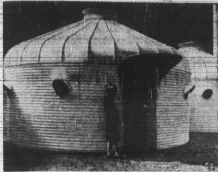
OUTSIDE—Siamese cylinders of corrugated steel—suggested for defense housing, evacuation buildings, barracks or bomb shelters can accommodate 24 people in double-decker bunks or family of six.
