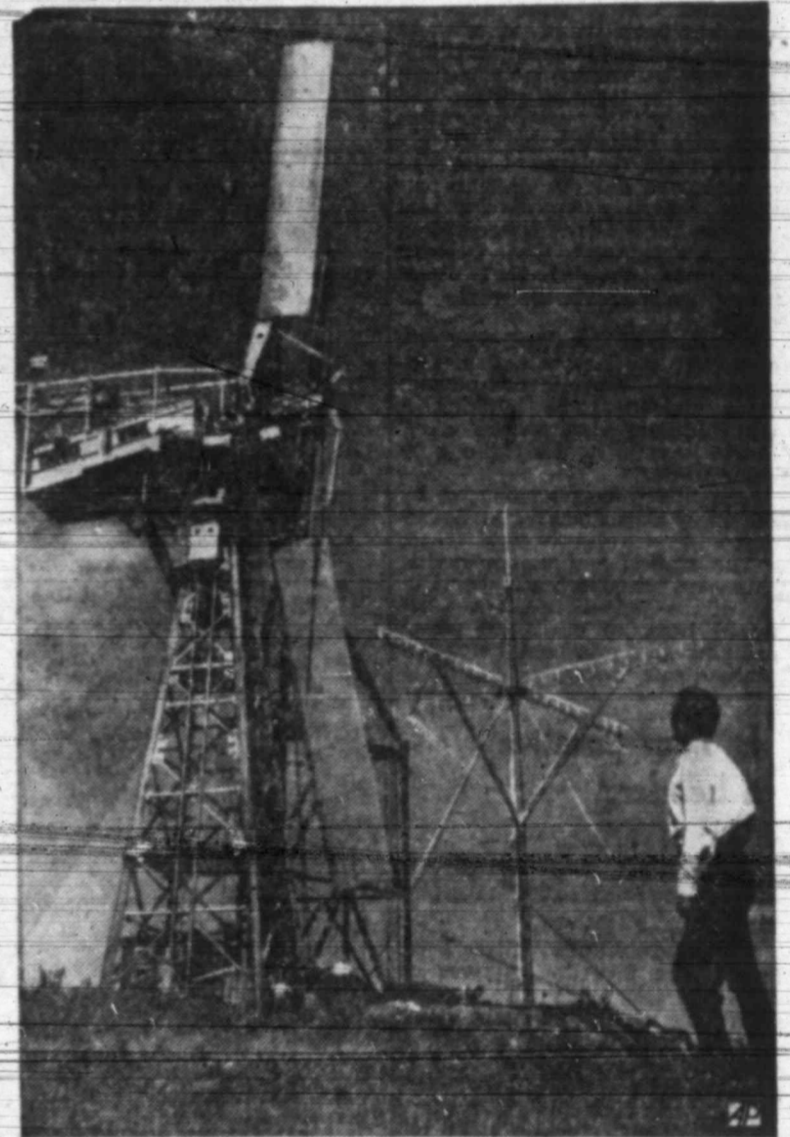
ANY WINDS TODAY? —Atop Grandpa's Knob, a 2,000-foot mountain at Castleton, Vt., this windmill whirs around, the second of its two 32-ton, 80-foot stainless steel blades having been recently installed. The windmill is designed to generate 1,000 kilowatts of electrical power, according to its designer, Palmer Casslet Putnam (above) of Boston.
