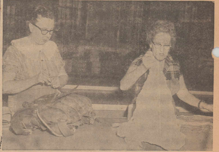
FOR SAFE LANDING —Workers in the base parachute shop constantly work with parachutes to make sure safe landings occur in case of bail-out. Inspections are made every 10 days, whether chutes are used or not, and every 60 days each parachute is thorough checked-out. Here Mrs. Thelma Williams seals a chute and Mrs. Maude Van Gundy starts repack of an SA-17. (Photo by Perez).
