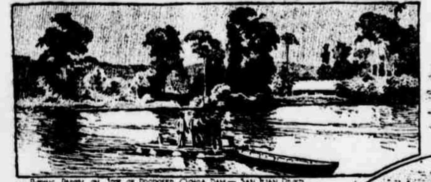
WORKING PARTY ON SITE OF PROPOSED CANAL DAM—SAN JUAN RIVER
