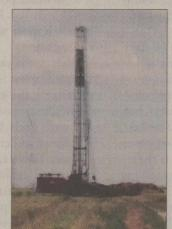
The rigging is up to begin drilling the first of two new water wells west of Lockney and just south of US Highway 70. Drilling, weather permitting, will take about three days per well. Once trenching, laying the pipeline, upgrading existing equipment and passing state testing is completed, the new wells should be added to the existing city water sources by September.
