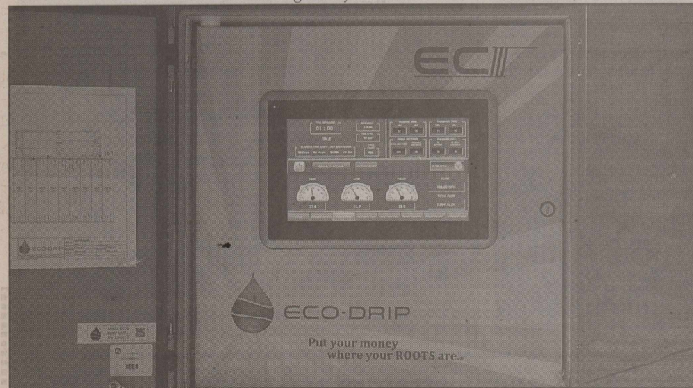
ECO-DRIP IRRIGATION systems are technologically state-of-the-art delivering fertilizer within the drip system. Frerich's controllers were simply programmed lawn sprinklers, but today, the controllers function in a computerized world with farmers having access to the system and its outputs on their smartphones.
