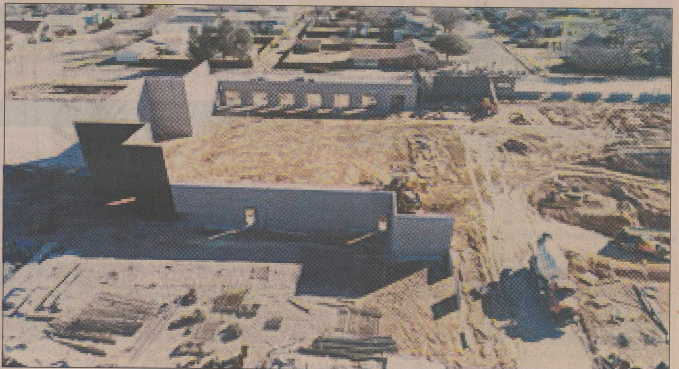
Shown are the exterior walls of the Auditorium.
