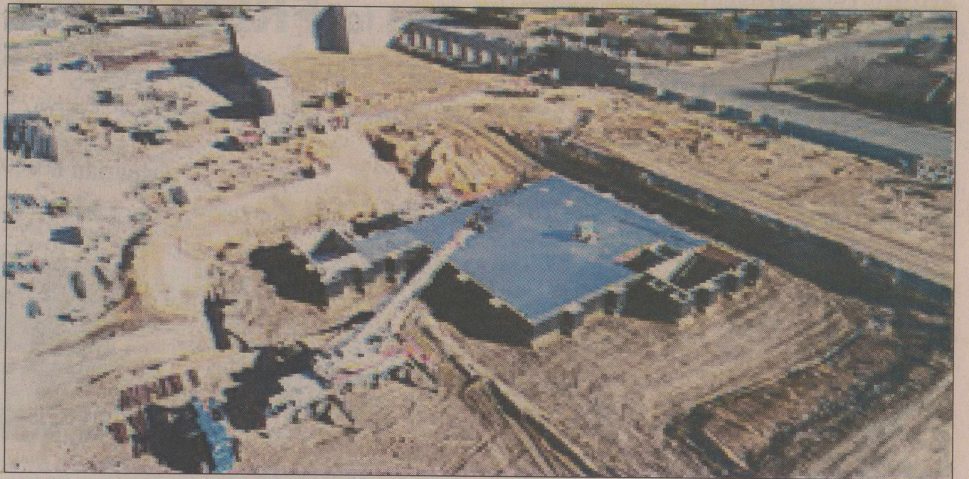
Shown is a view of the completed basement roof.
