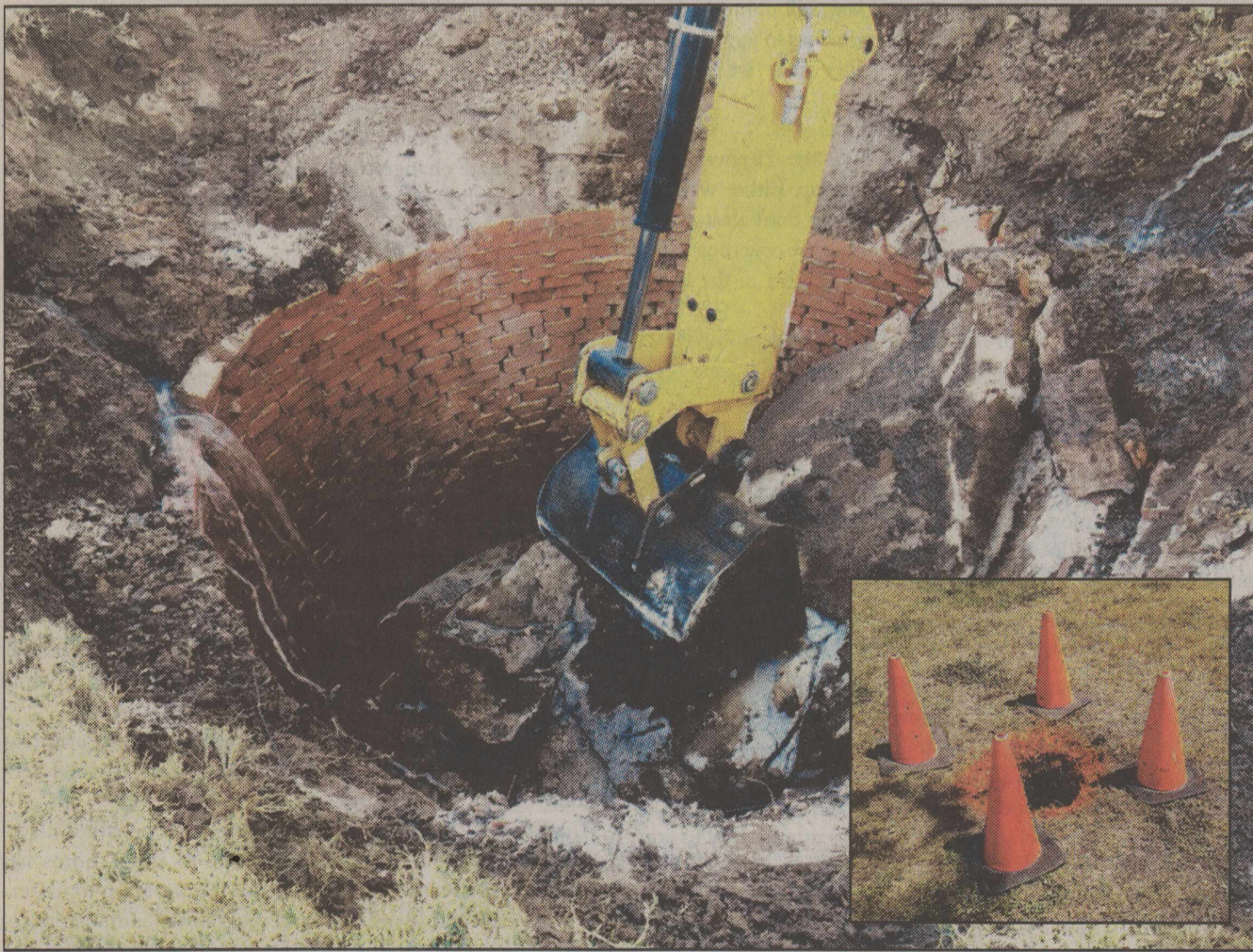
A small sinkhole (inset) in the courthouse lawn collapsed, revealing a hidden room underneath which was most likely a cistern at one time. County employee Tracy Webb used a backhoe to open up the area, a 20 foot wide round room, before filling it in.
