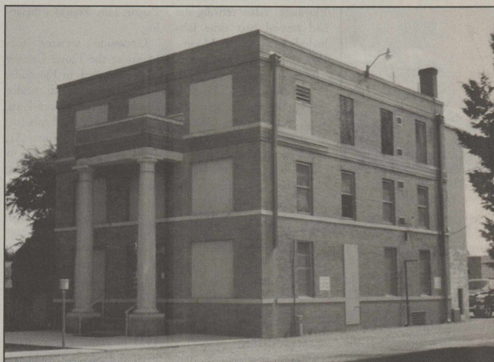
In the July county commissioners meeting there was a public hearing about the demolition of the Old Jail, and no one from the public attended. The court is moving forward with steps to demolish the building.
