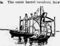
NOT ALTOGETHER A SUCCESS ing the interior stationary. It can be steered, but very poorly. Sails can be attached, but progress is very slow. Capt. Beckman fully believed that he could reach Rockland safely, but it is
