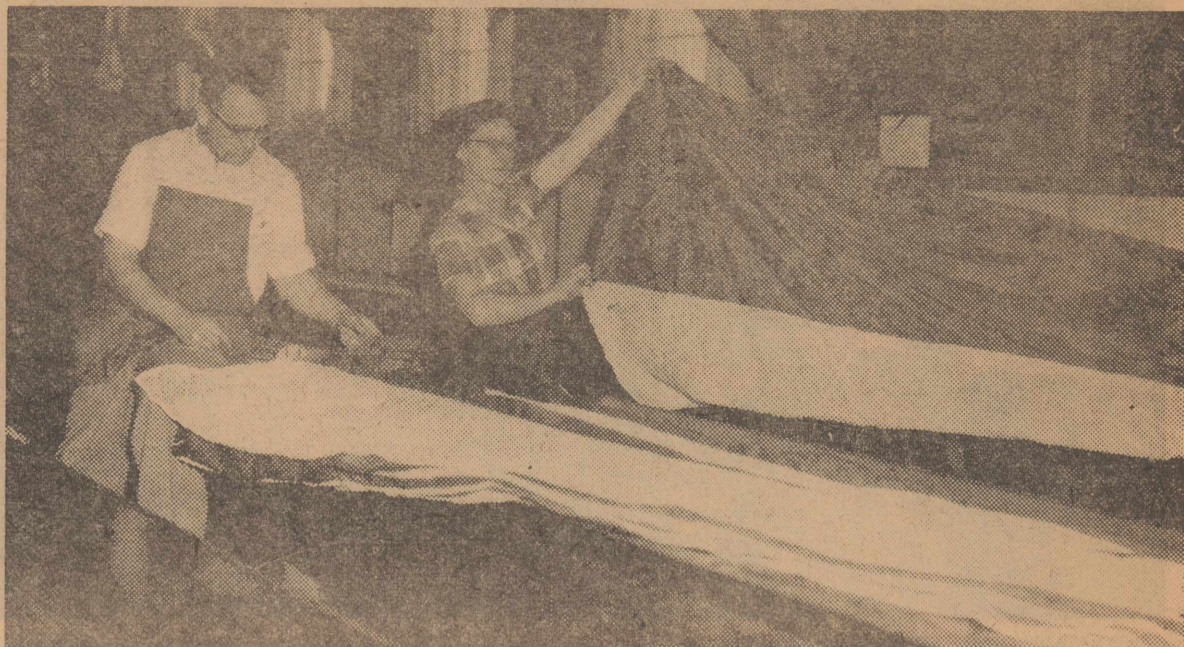
PARACHUTE RIGGERS — Mrs. M. Turner and Mr. R. Brag string the chute on these two-44 foot tables when they repack the parachute. This entire operation requires 45 minutes. After being repacked, the chutes are sent from here to the fabric workers who repair and restitch harness and bindings.
