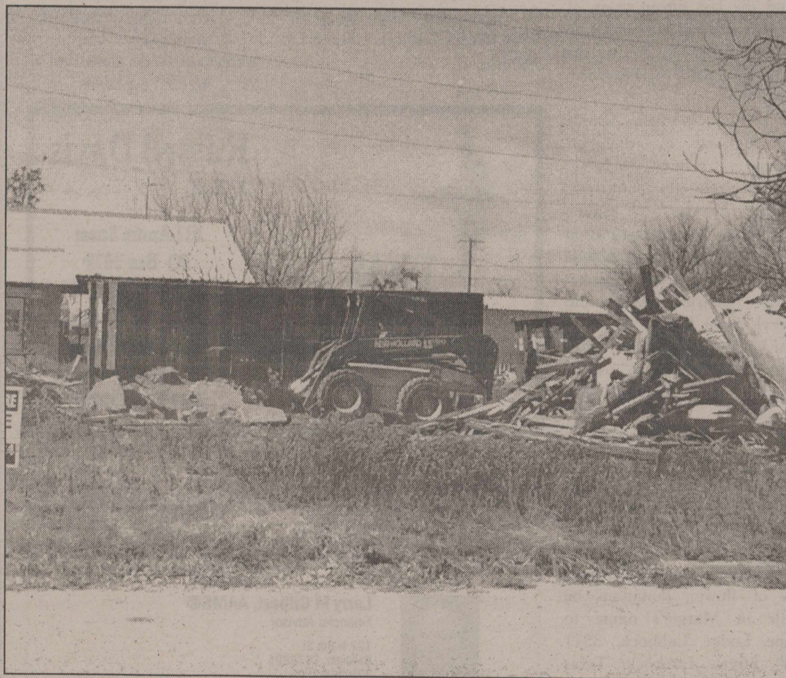
Bronte Demo! Bryan Swecker and Reese Braswell put in a couple of days of work last week and filled two large dumpsters removing the dilapidated house in Bronte on North Washington Street across from the water treatment plant. This is the first of many dilapidated houses Restoring Bronte Foundation and area volunteers have targeted for demolition in their quest to improve Bronte.
