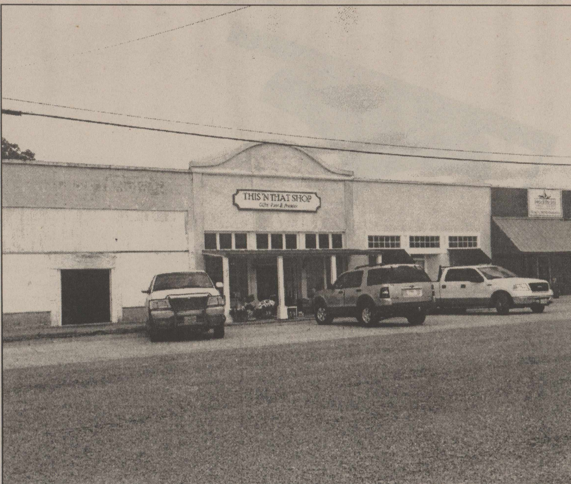
Storm Clean-Up! Cloudy skies had not yet given way to drying sunshine as Leta and Cyndi Caston began the clean-up from Monday night's storm. Water ran in the back of This 'N That Shop on Austin Street in Robert Lee. Fortunately, Leta's building next door remained dry and they were able, with assistance, to move much of their inventory. Leta says to be ready for a big upcoming "Water Sale"!
