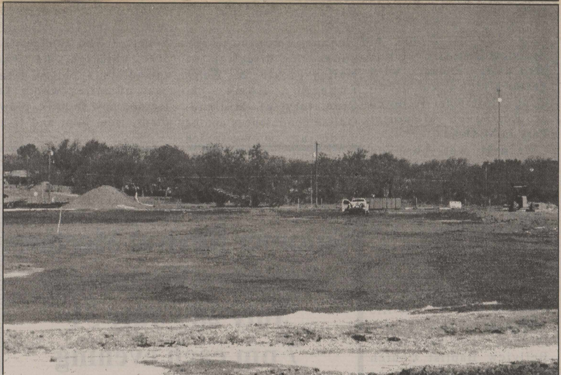
What a difference a couple of months make! The bottom photo is a look at the Robert Lee High School stadium the first of May. The top photo was taken last week. The new stadium should be completed by August 1st and the community can get a closer look when they attend the RLHS 2014 Project Graduation Hot Dog Supper the evening of August 15th. The first varsity game in the new stadium is set for 7:30 pm Friday night, August 30, 2013, between the Robert Lee Steers and the Longhorns of Meeteetse, Wyoming.
