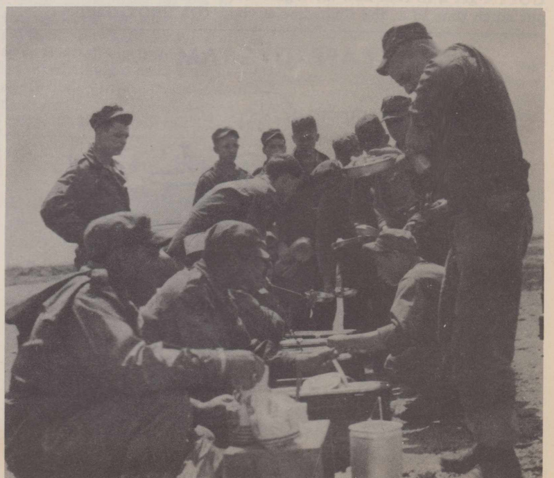
Engineers of Company A, 809th AF Engineer Battalion, pause for chow after a morning's work of clearing vegetation from the runways and taxiways at the Abernathy Auxiliary Field. This is one of the many jobs the enginners will accomplish before moving on to other Training Command Bases or returning to their home station. (Photo by Cpl. Massie)
