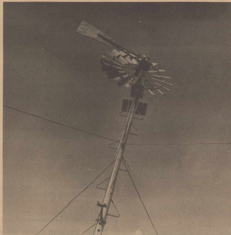
THIS IS WEST TEXAS --- Oops, a one-legged windmill. This is West Texas but sort of a freak of a windmill tower. The windmill is located just north of the Phillips plant on the Denver City Highway on the ranch land and farm land of N. S. Woods. The four guy-wires anchor the one legged tower to hold it in its upright position. It is an Aermotor (not air and not aere motor as some of you tried to tell me; I don't care if you did live on the farm where they had one of these). The mill was built in Chicago, Illinois and the one leg sets at a slight angle to allow the lift rod to run at a straight line from the mill to the well. With the fan setting next to the blades the windmill was cut off at the time the picture was made. Other interesting things about the one legged mill is the ladder, also the two braces that the succor rod goes through.
