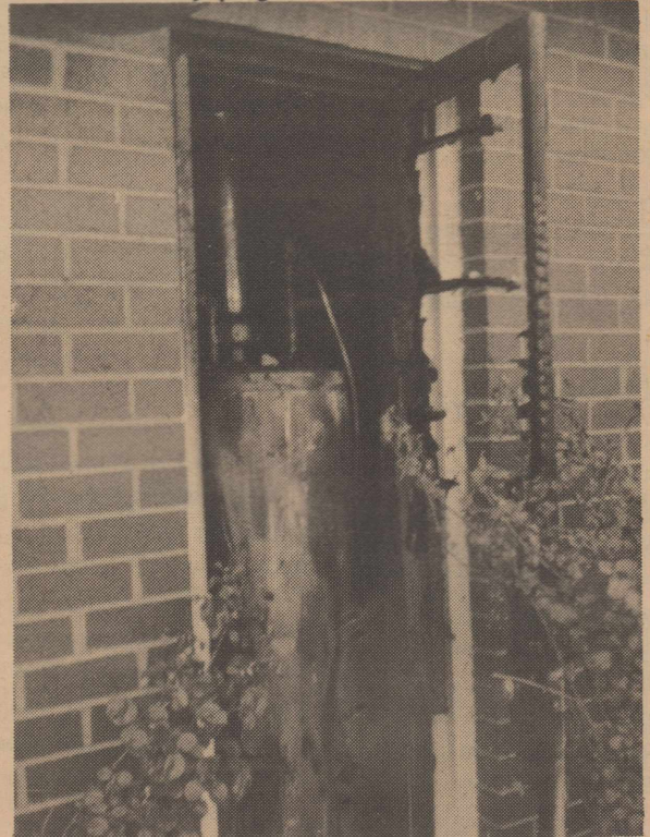
The Seminole Volunteer Fire Department was called to 401 S. W. 18th at 6:25 p. m. Monday to a fire in a hot water heater closet opening to the outside at the home of Mary Jo Kennedy. A passing motorist, Tommy Montandon, extinguished the blaze with a garden hose after his wife saw the flames coming from the house. It was reported that the fire was caused by leaking gas.
