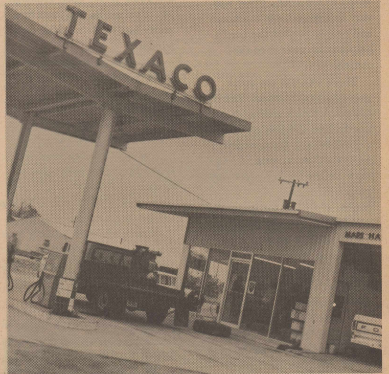
Home of Marshall's Tire Repair, 501 East Lamesa Highway.
