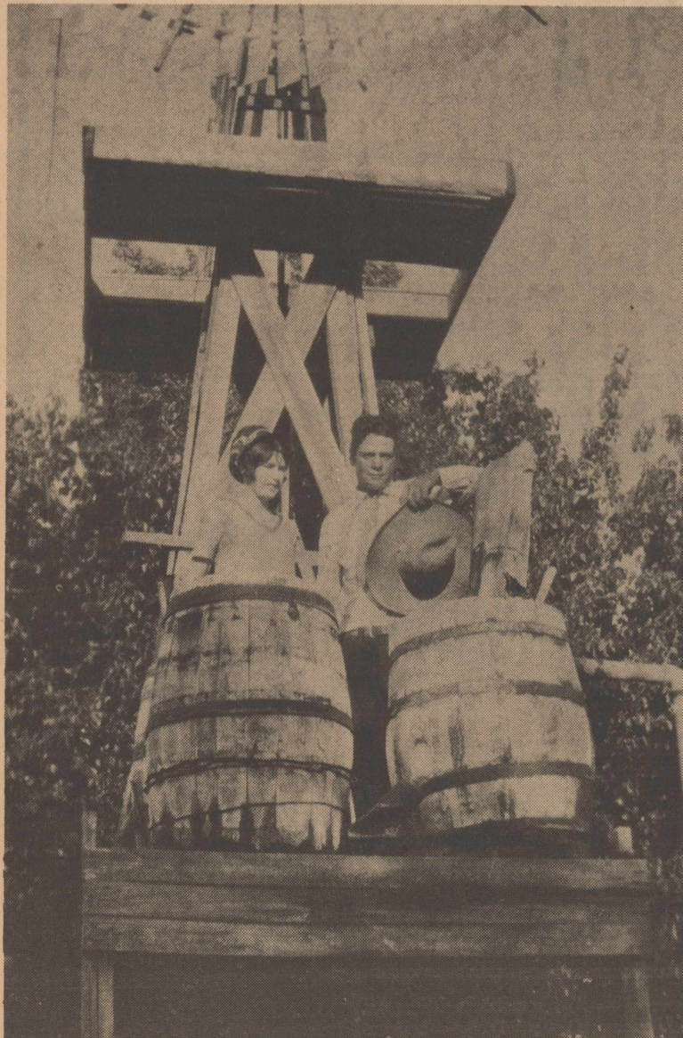
IT WAS SUNDAY AFTERNOON, IT WAS SPRING, AND IT WAS PICTURE TAKING TIME. JOHNNY SPARKS AND BETTY (MC-CLESKY) THOMPSON AS THEY HAD THEIR PICTURE MADE ON THE OLD AUSTIN PLACE ON S.W. AVE. G. THE WATER SUPPLY CONSISTED OF TWO 55 GALLON WOODEN BARRELS ON A STAND SUPPORTED BY THE WIND TOWER. NOTE THE OVERFLOW PIPE AND ESPECIALLY THE OLD ECLIPSE MILL. THE YEAR?—A GOOD MANY AGO.
