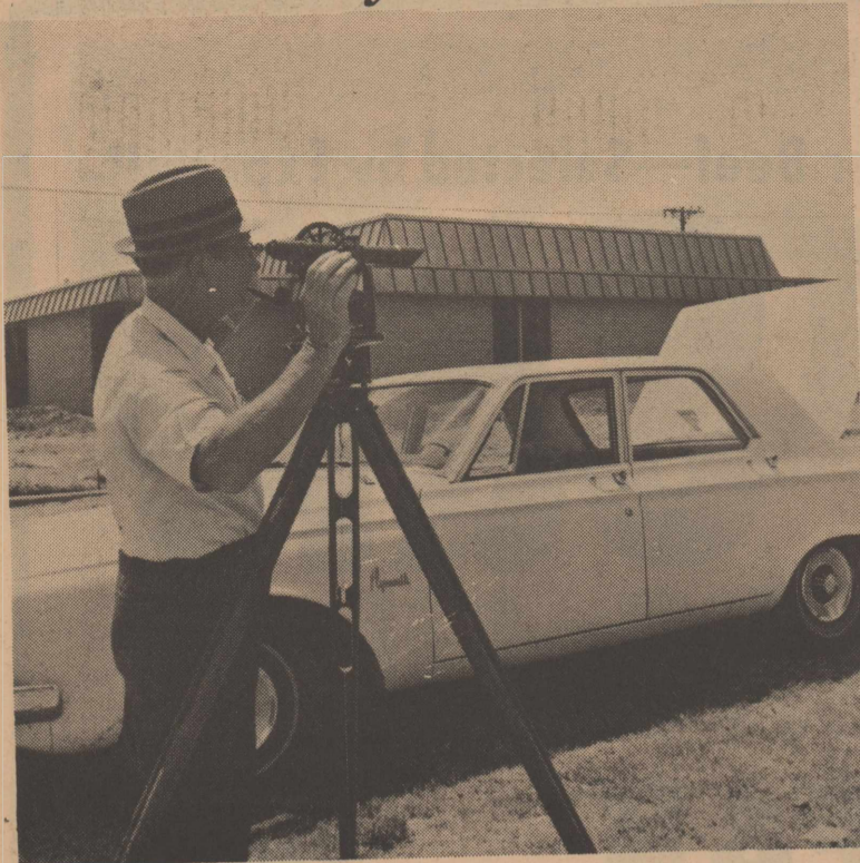
C.A. Tubbs, Consultant Engineer for the City of Seminole, is surveying and running elevations on N.W. Ave. B. for curb and gutters. He and his surveying crew have finished everything west of Main and south of S.W. Ave. G. He hopes the paving contractor will soon be on the street paving project. In the picture he is giving hand signals to Danny Ammons from Seagraves as he is setting the stake.
