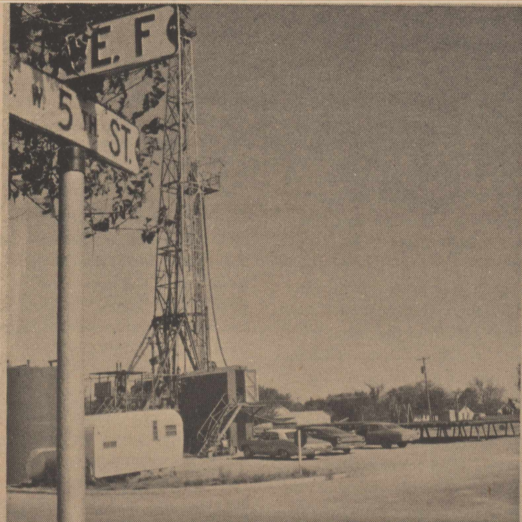
The oil well rig drilling at Ave. F. and S.W. 5th Street is not for oil. It is to be used by the Amerada Petroleum Company as an water injection well for the water flooding program. The Cactus Drilling Company owns the jack knife rig. Ben Morefield, driller, and Bobby Joe Murphy can be seen working in the derrick. Neighbors have asked sight seers to please be careful in the area and watch where they're driving or stop to watch the drilling rig.
