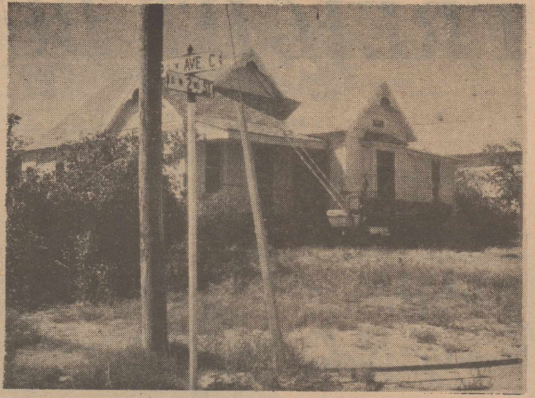
THE RESIDENCE OF SAM MALONE, "TOP" HURD, TOM ROSS, BERT ANCELL, AND OLAN LOCKER. THE HOUSE WAS LOCATED ON AVE. C AND 2ND, ST., S.W. ACROSS THE STREET FROM THE GAS OFFICE, BEHIND FOREST LUMBER COMPANY. THE HOUSE WAS 40' X 54'. THE CEILINGS WERE 9'. THE ORIGINAL PART OF THE HOUSE WAS 'BOX'. PART OF THE FLOORS ARE STILL PINE, OTHERS HAVE BEEN COVERED WITH OAK.
