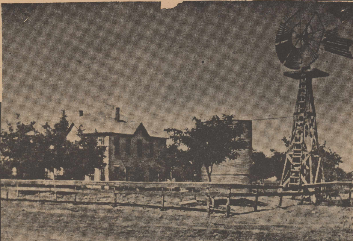
Court House, Gaines County, Seminole, Texas.
