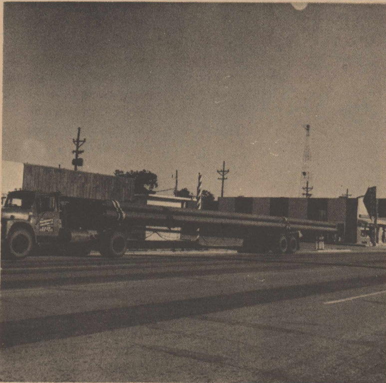
This truck with 11 stalks or pieces of 16" pipe is headed for the gas line being built for Shell by the Great Plains Construction Company. The pipe averages 78 inches in length and some measure up to 85 inches. PARKED ON OUR HIGHWAYS LAST FRIDAY MORNING, H&D Food can be seen in the background.
