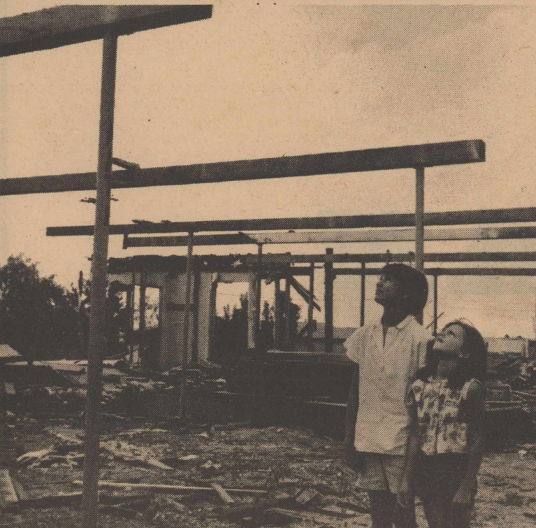
Annie and Wanda Brasher, daughters of Mr. and Mrs. J. E. Brasher, look up at the remains of the two-story, 4 apartment building at 304 S. W. 16th St. The Jess O'Neals and the J. E. Brashers, and the Crespin Mejias and other Seminole residents are rejoicing that the final remains of the building are being moved.
