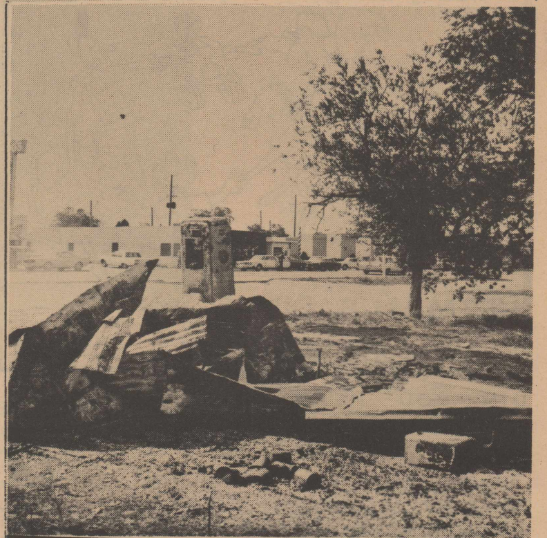
Just a few pieces of tin, a commode tank and an old gasoline pump is all that remains of the old station building at 617 S. Main.
