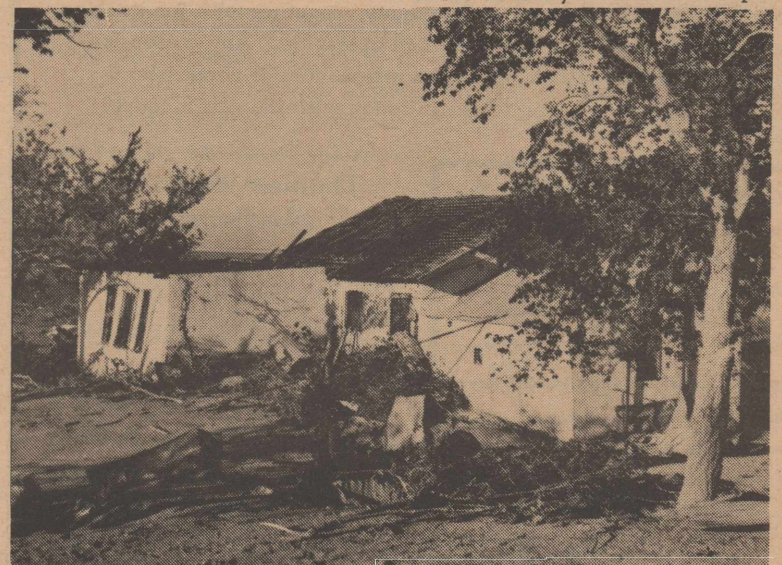
Debris and the unroofed farm house seven miles northwest of Seminole can be seen after the twister last Saturday.
