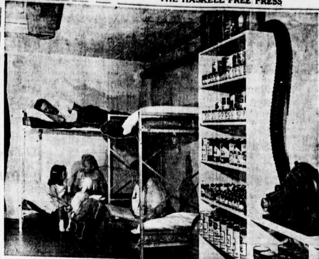
FALLOUT SHELTERS are the best way for rural Americans to protect themselves from a massive nuclear attack which could unleash dangerous radioactive fallout throughout the country. Some of the shelters recommended by the Office of Civil and Defense Mobilization are not as elaborate as this one, which includes an auxiliary generator and an electric air filtering and ventilating system. However, all recommended shelters should include the basic features shown here—a place to sleep; food, water and medical supplies, and at least eight inches of concrete or an equal weight of other materials for shielding the shelter against fallout. Free designs may be obtained by writing to OCDM Rural Civil Defense, Battle Creek, Mich. (OCDM Photo)
