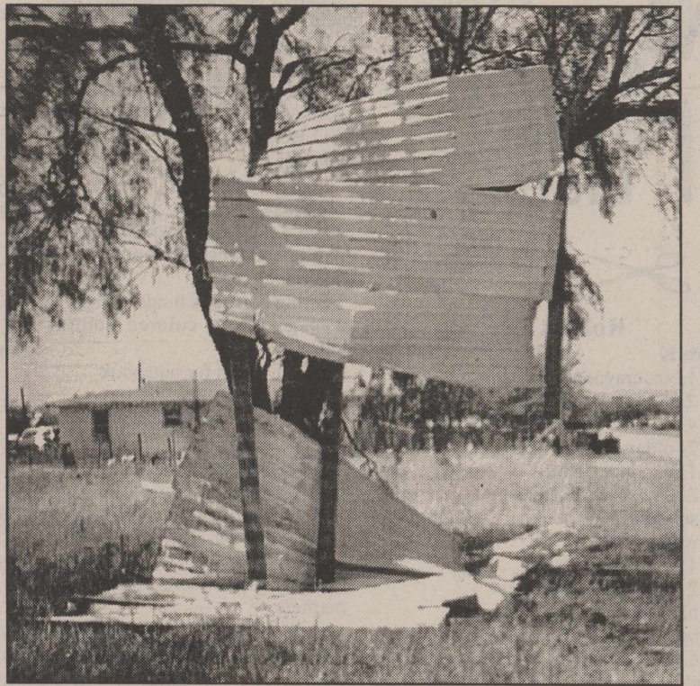
Robert Lee Storm Damage! Bud Thompson took these pics of the damage done during Saturday night's storm in Robert Lee. The quick moving cell tore a strip through town with its high winds and driving rain. This trailer at 5th and Alamo had part of its roof relocated to a nearby tree.
