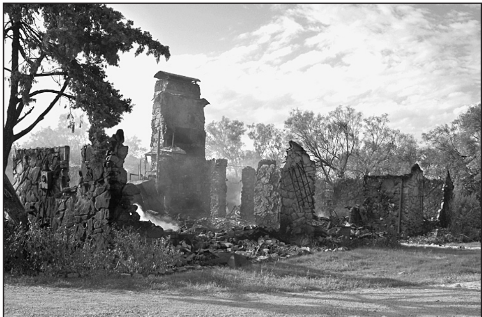
HOUSE DESTROYED —The Haskell Volunteer Fire Dept. was called to this house fire at approximately 1:30 a.m. on Tues., Aug. 10. The house is located approximately 3 miles south of Haskell on Hwy. 277. Cause of the fire is under investigation.
