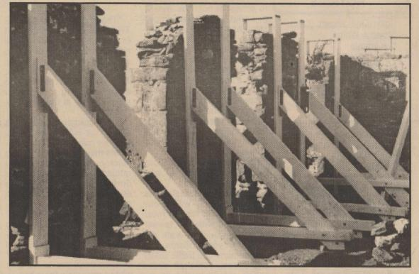
The walls of the barracks at Fort Chadbourne have had bracing installed to guard against further deterioration.
