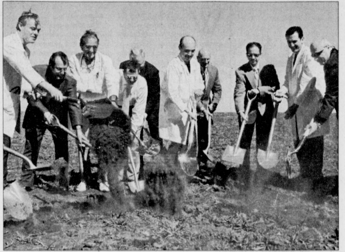
FUTURE HEART HOSPITAL doctors and community leaders break ground at the future hospital site Tuesday morning. The center, located north of Loop 289 and west of Quaker Avenue, opens in December.
