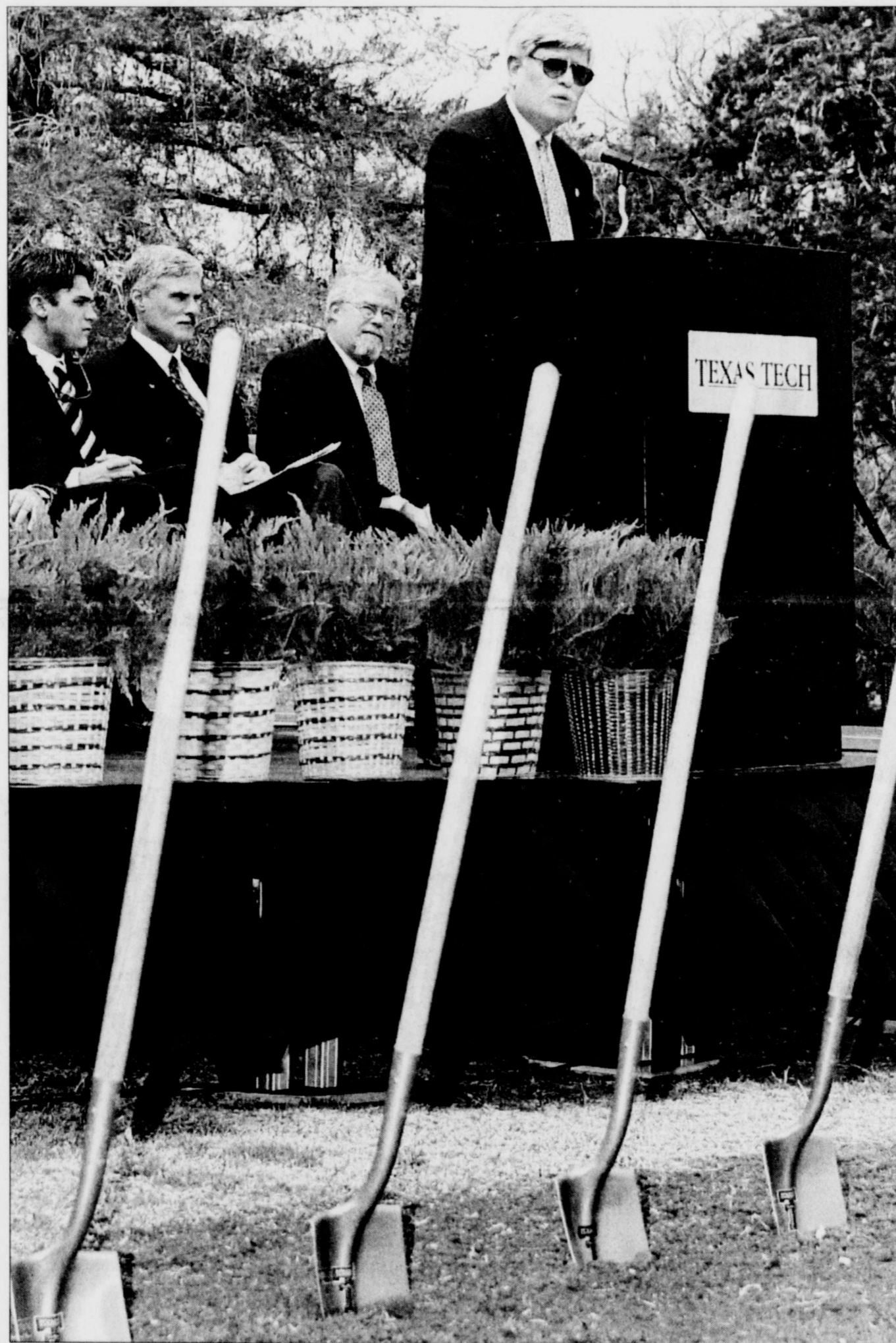
OUTGOING PROVOST JOHN Burns speaks about the new Experimental Sciences building at the building's groundbreaking Thursday. The building will be located north of the Biology building, where a portion of the R-2 lot is located.
